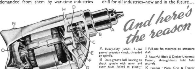
minimizes wear, ensures spindle accuracy. C Splined mounting of spindle gear increases strength, facilitates inspection, reduces noise,
